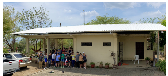
New Roof at La Boquita!
